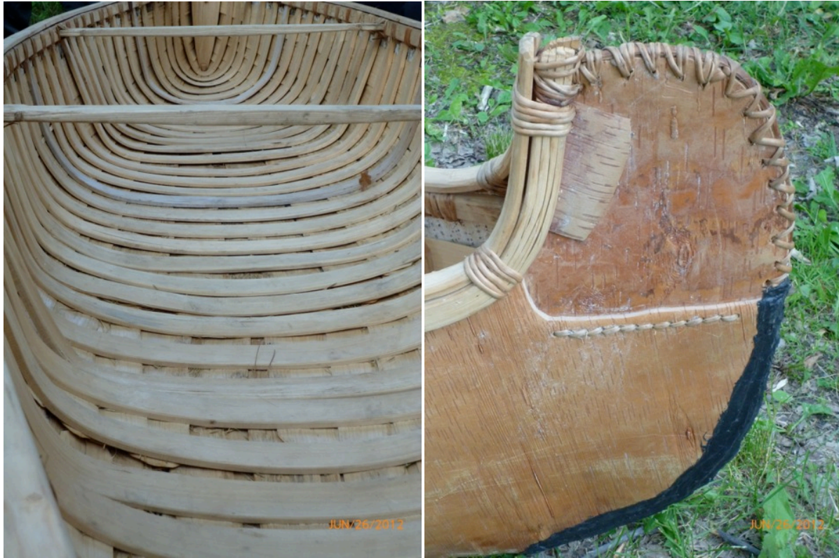
Figure 56. Cedar ribs over cedar planks interior detail (left). Spruce root lacing detail (right) of Jones' birch bark canoe. Courtesy Kevin Slivka, author.
