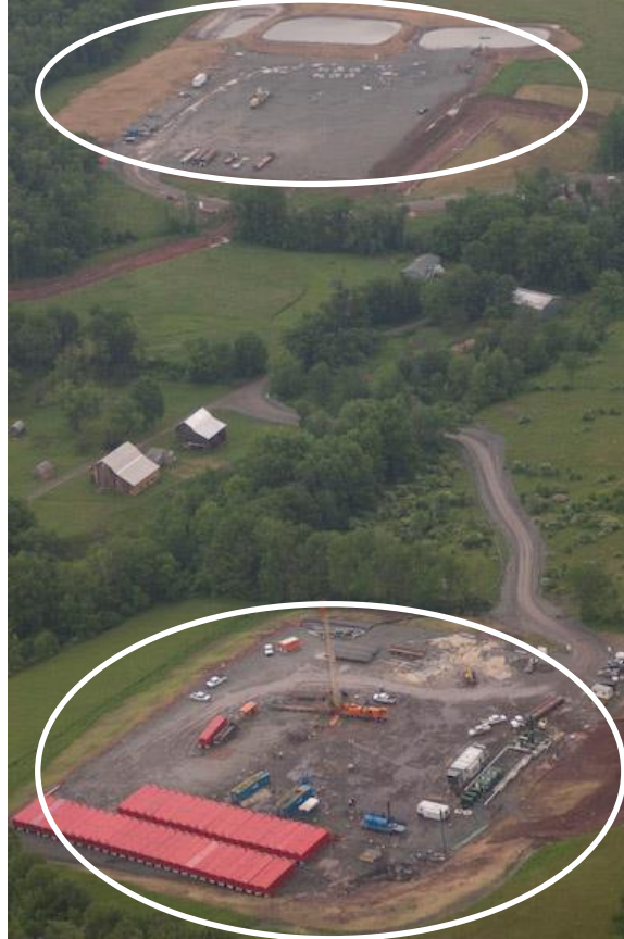
Figure 3. Two Marcellus Shale well pads, shown above outlined in white, in Bradford County, PA. The pads have been surfaced with crushed limestone and are both in the active development stage (MSETC 2010). The upper well pad has a number of water storage ponds located along its upper side.
