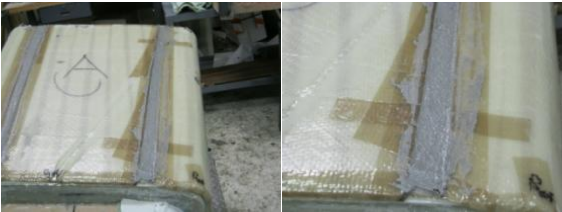
Figure 3-38. Super Ceramic Repair Putty application.
