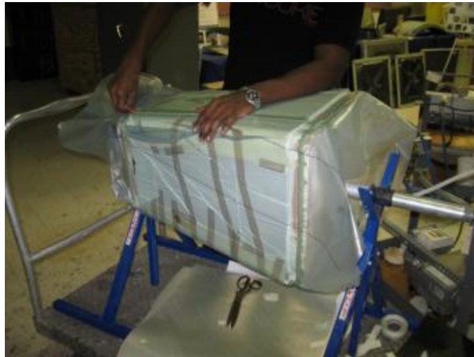
Figure 3-16. Spar under vacuum in preparation for de-bulk/cure
