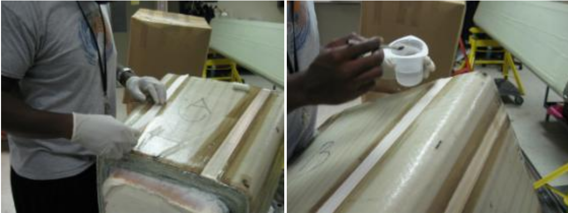
Figure 3-45. Syntho-Glass with Caul Blocks
