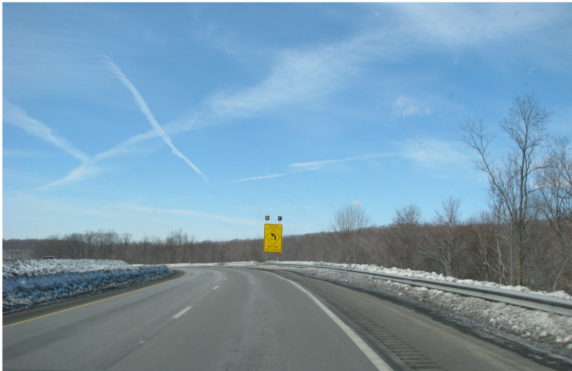
Figure 2 – Example of Data Collection Site in West Virginia
