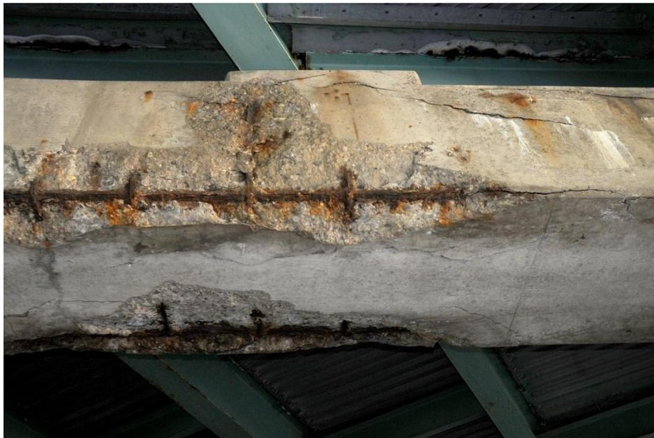
Figure 3-27: Corrosion of steel reinforcing bars in concrete (Courtesy of Matco Services, Inc.)
