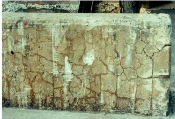
Figure 2-1: ASR crack manifestation (courtesy of FHWA)
