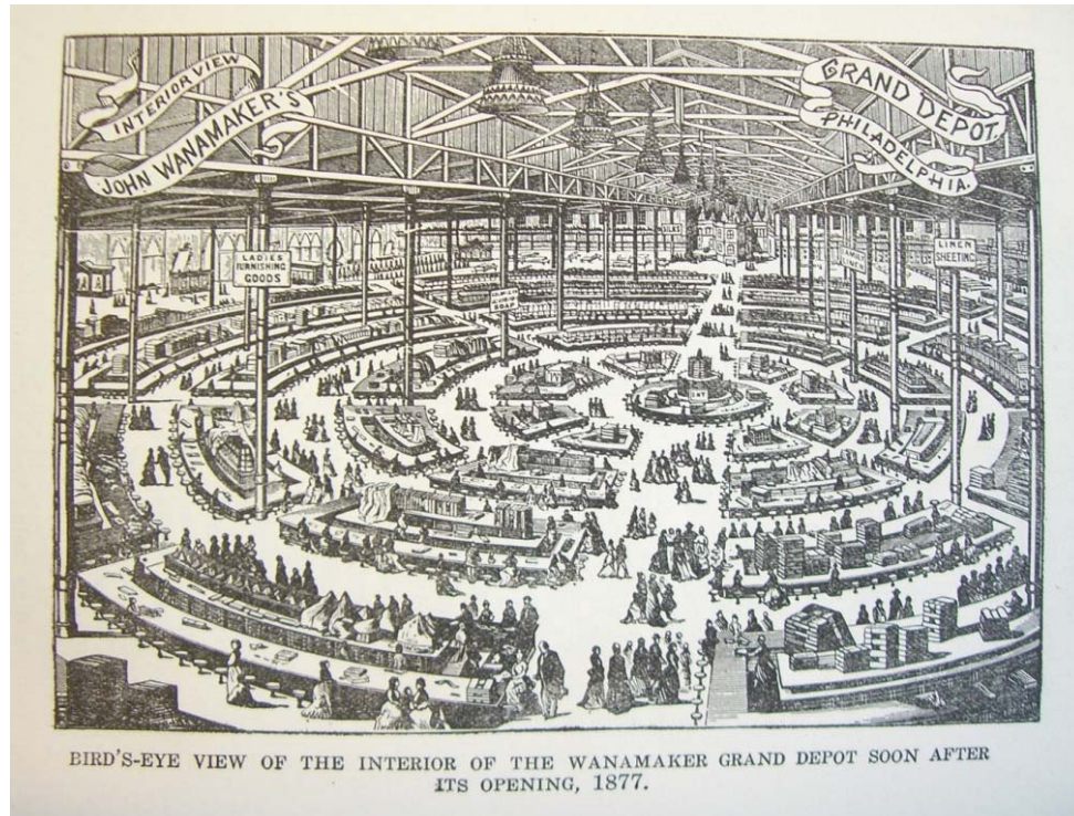
Figure 3.3 Interior of Wanamaker's Grand Depot, 1877 (Source: Wanamaker, 1911:following 56)
