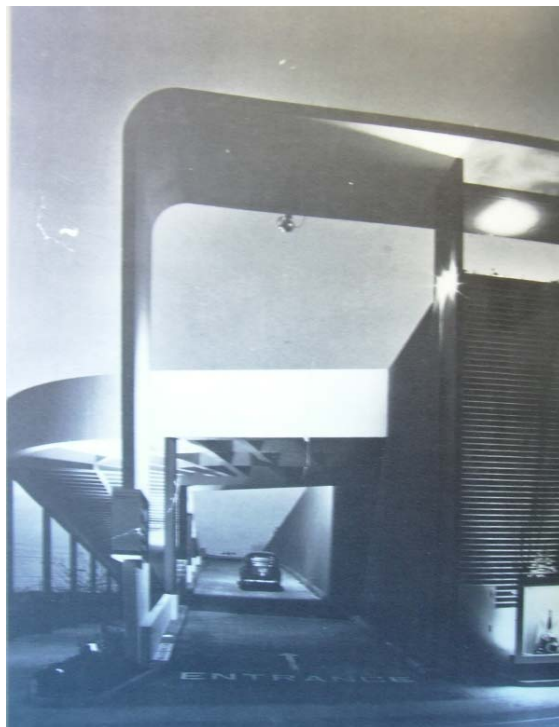
Figure 5.5 Milliron's, ramp to parking deck (Source: Hardwick, 2004:98)
