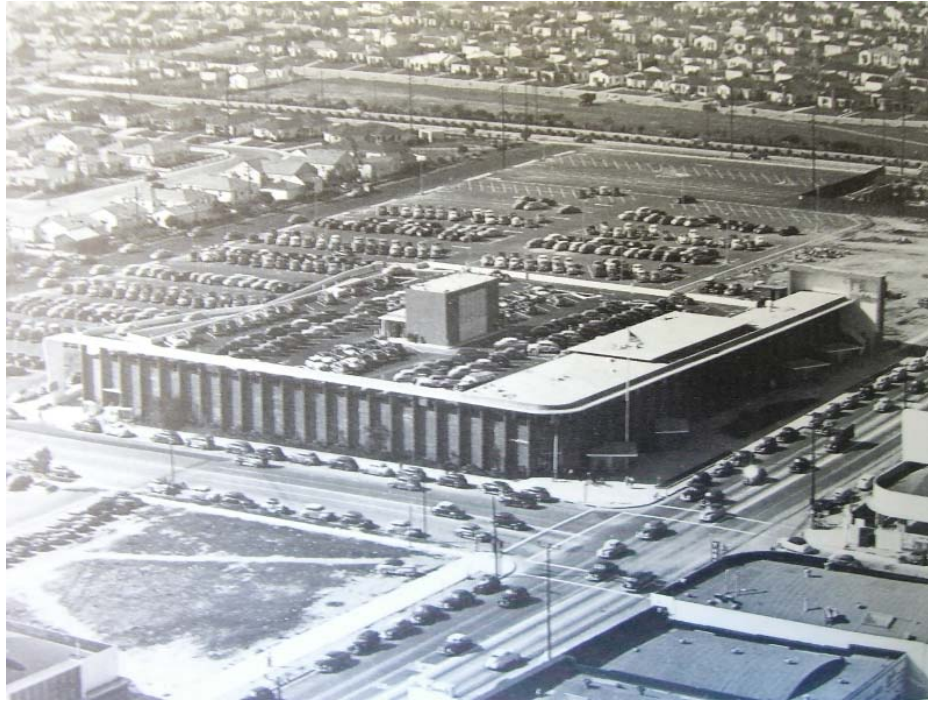
Figure 5.4 Milliron's exterior, showing rooftop parking deck (Source: Hardwick, 2004:97)
