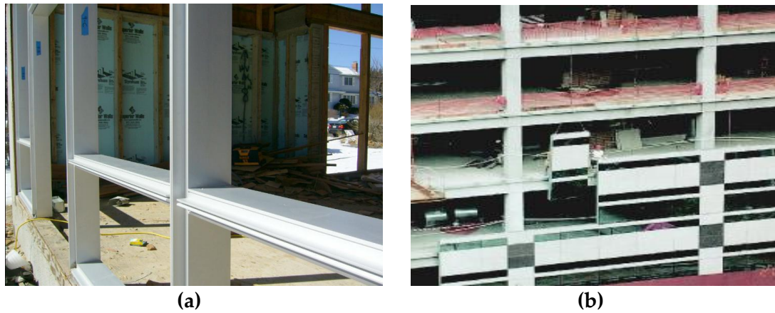
Figure 2.2: Comparison between (a) stick-built and (b) unitized CW systems ( www.livemodern.com , www.archsd.gov.hk )
