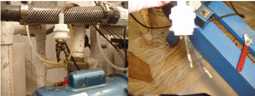
Figure 5.7: Thermocouples before and after cleaning off
