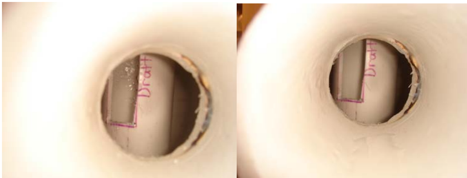
Figure 5.3: Picture through Overflow Line Hole
