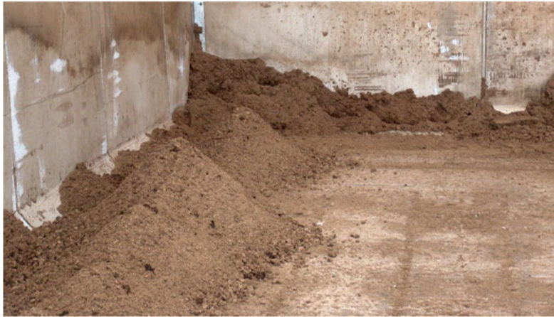
Separated solids drying on the slotted floor in the bedding storage area
