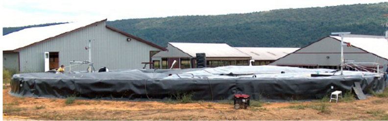
Digester with flat cover
