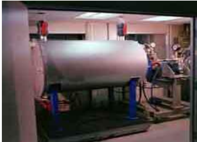
Figure: 3 ANAEROBIC DIGESTER TANK DOE
