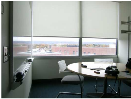
Fig 2-1: An interior translucent fabric shade and automated shade control application (Photo credit (right): Lutron™).
