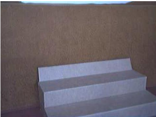
Figure 4: Camera Image of Stairway
