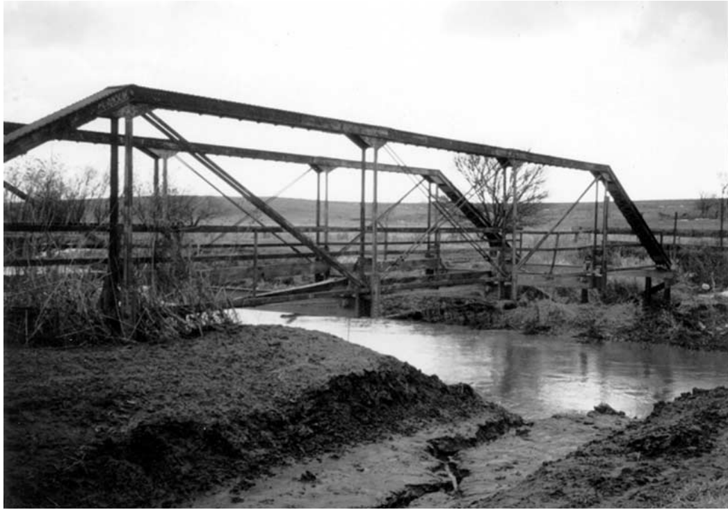
Figure 3-1. Rock Creek Bridge
