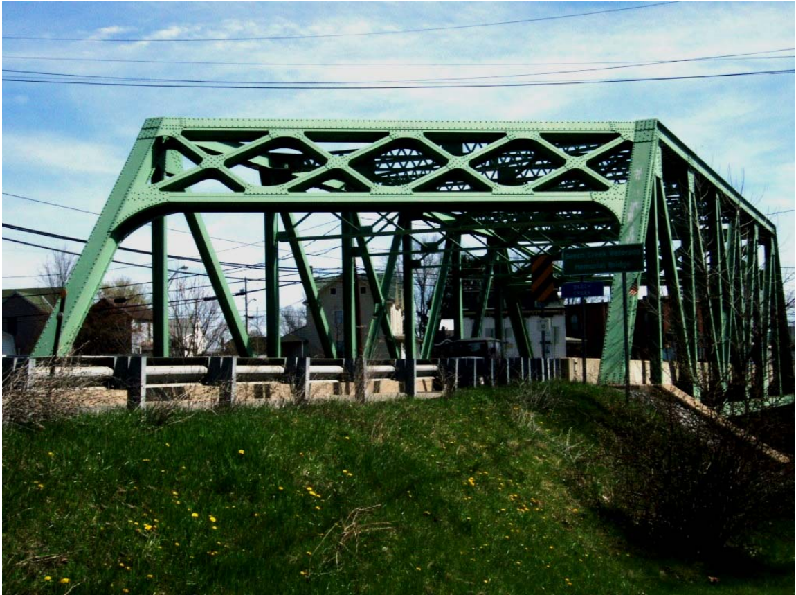
Figure 3-4. Beech Creek Veterans Memorial Bridge
