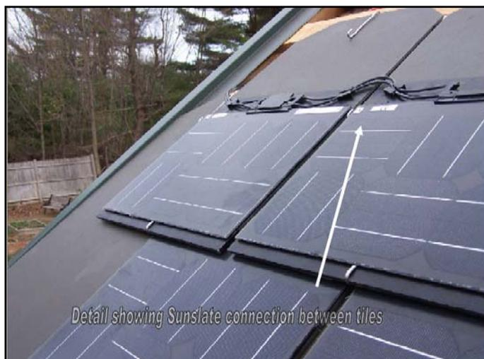
Figure 5-3 (a) Wiring details between slates on walls
