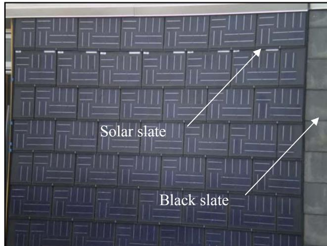
Figure 5-2: Image of the installation of solar slates
