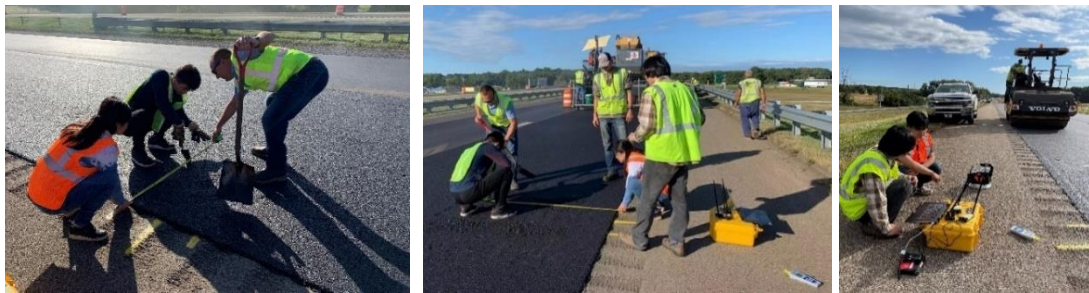
Figure 4-6 SmartKli ® installation and data collection in Indiana project
