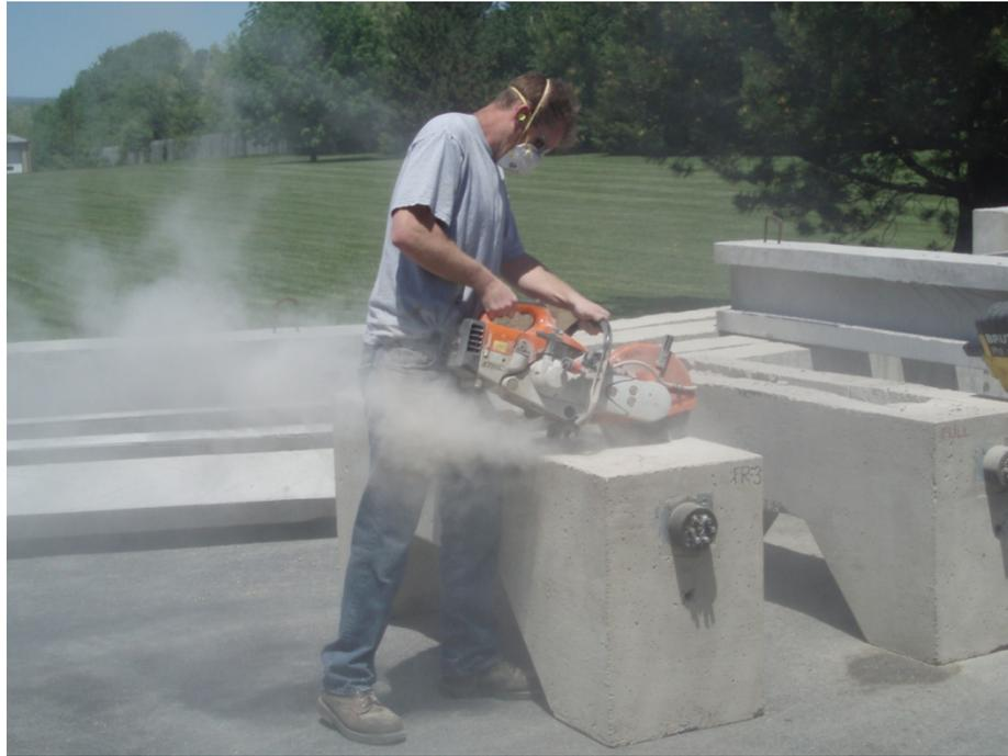
Figure H-4: Saw Cutting of Concrete Above Tendon and Anchorage
