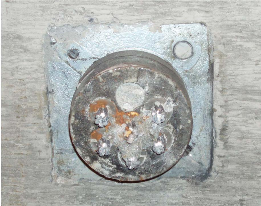
Figure 6-10: Strand Corrosion at Anchor Head Opposite to Grout Void
