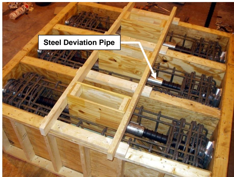
Figure 4-5: Photograph Showing Location of Steel Deviation Pipe
