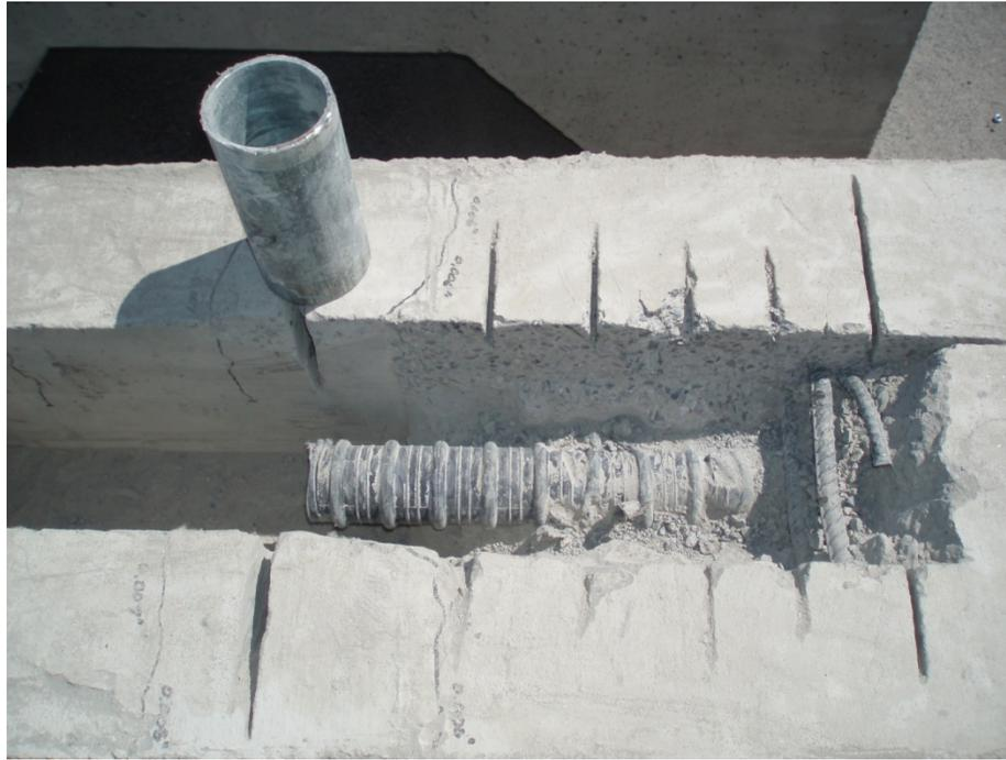
Figure H-3: Concrete Removed to Expose Tendon
