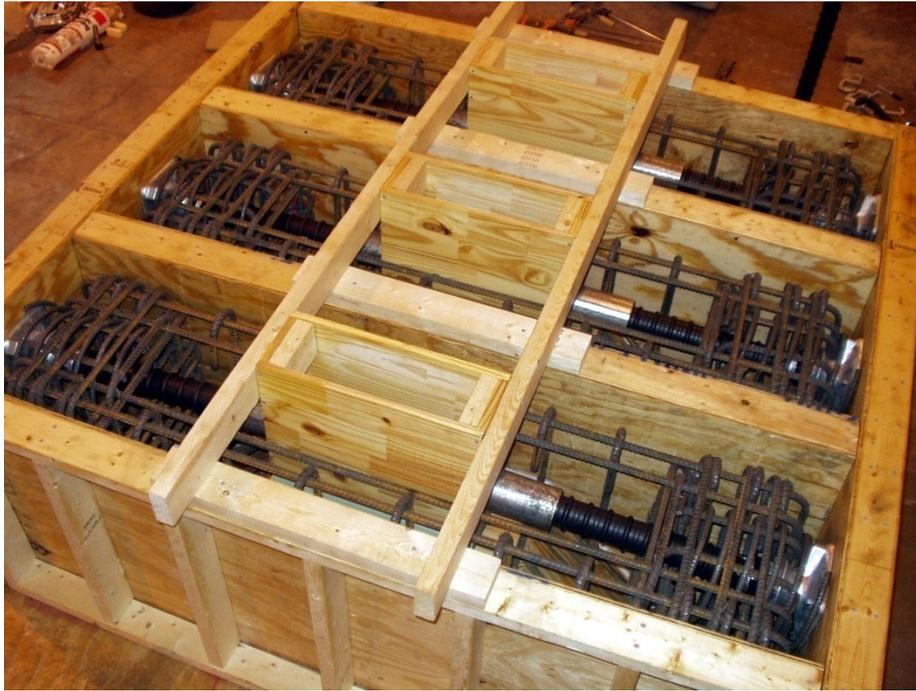
Figure C-4: Completed Specimen Setup Ready for Concrete Placement
