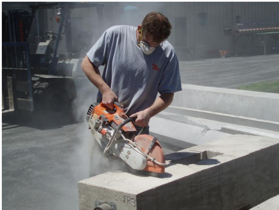
Figure H-2: Saw Cutting of Concrete Above Tendon
