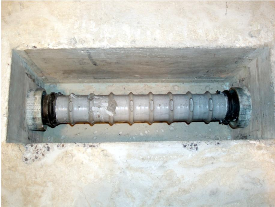
Figure 5-10: Exposed Grouted Tendon After Plastic Duct Removal
