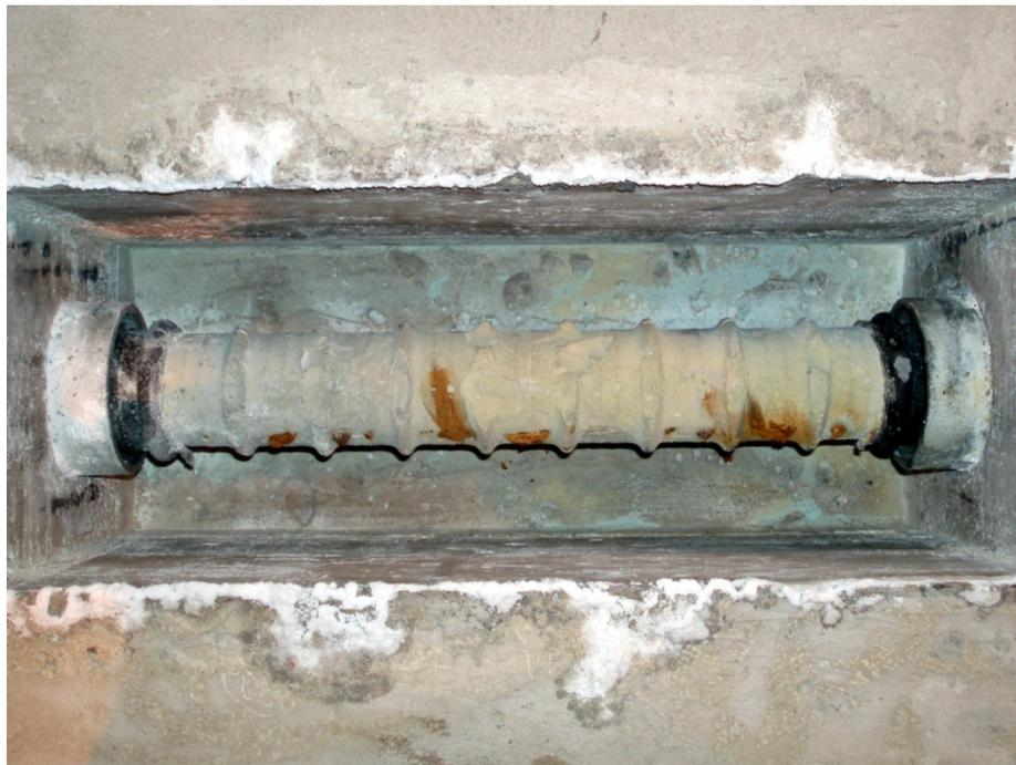
Figure 5-14: Exposed Grouted Tendon for GVC-1 Showing Signs of Corrosion
