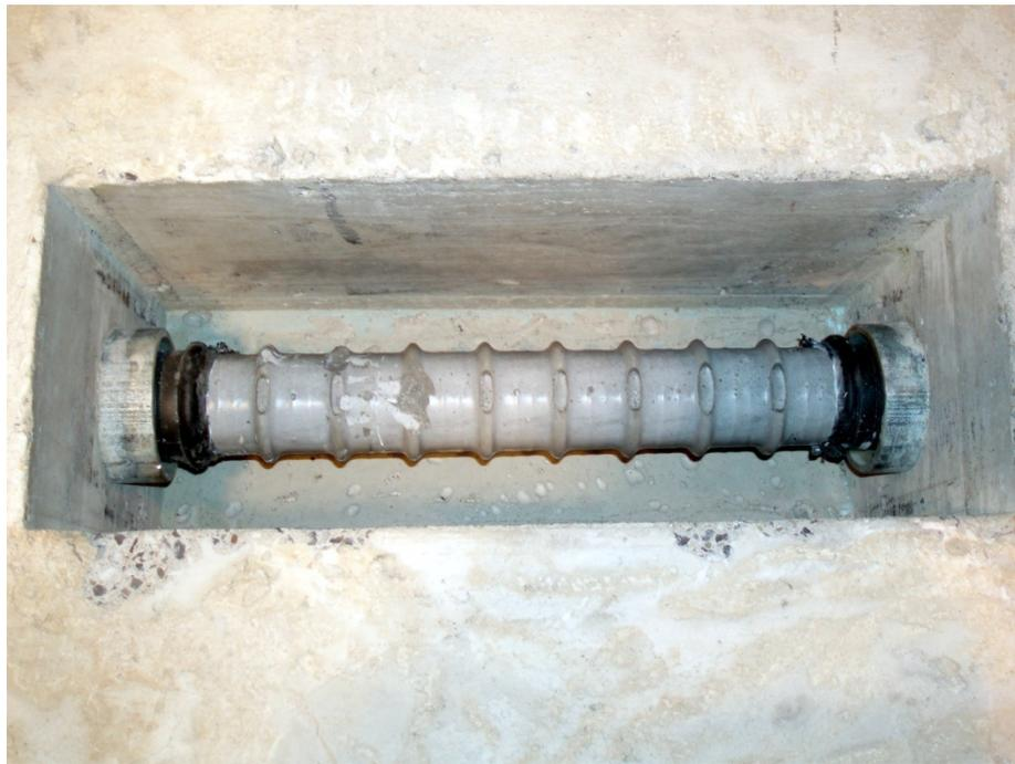
Figure 6-1: Exposed Grouted Tendon After Plastic Duct Removal for *In situ* Inspection
