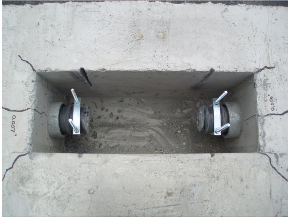
Figure H-1: Removed Center Portion of Tendon
