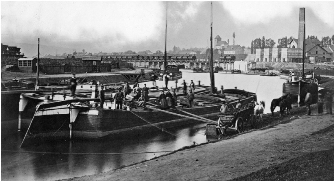
Figure 12 - View of the Mouth of the River Port Island, c. 1870's, Malstatt-Burbach. Elevated rail lines and coal chutes used to load barges along the northern edge of the harbor located in the background.
