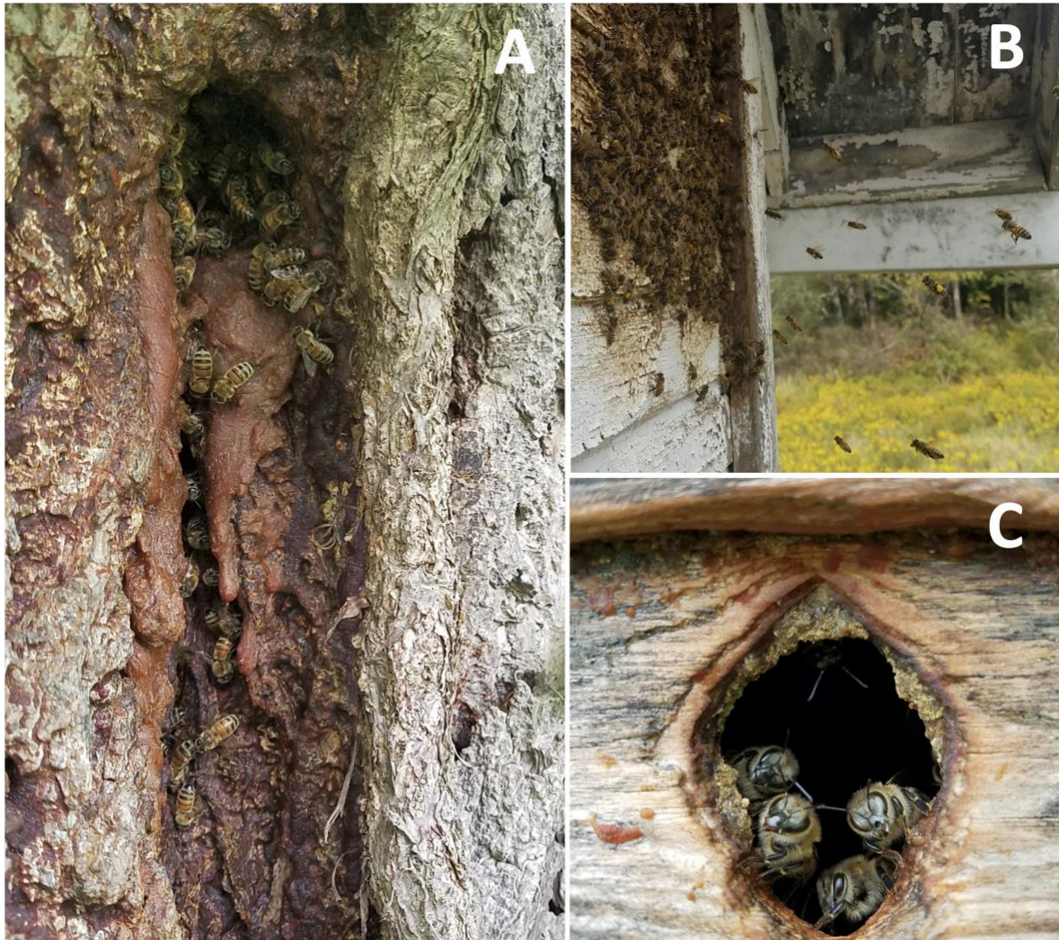
Figure 2.1: Cavities used by feral honey bee colonies included in the study. (A) Colony inhabiting a tree cavity with abundant propolis at the entrance of the nest in Saxonburg (PA, United States). (B) Feral colony nesting inside the wall of a house in New Bethlehem (PA, United States) (C) Entrance of a feral colony nesting in an abandoned shed in Harrison Valley (PA, United States).
