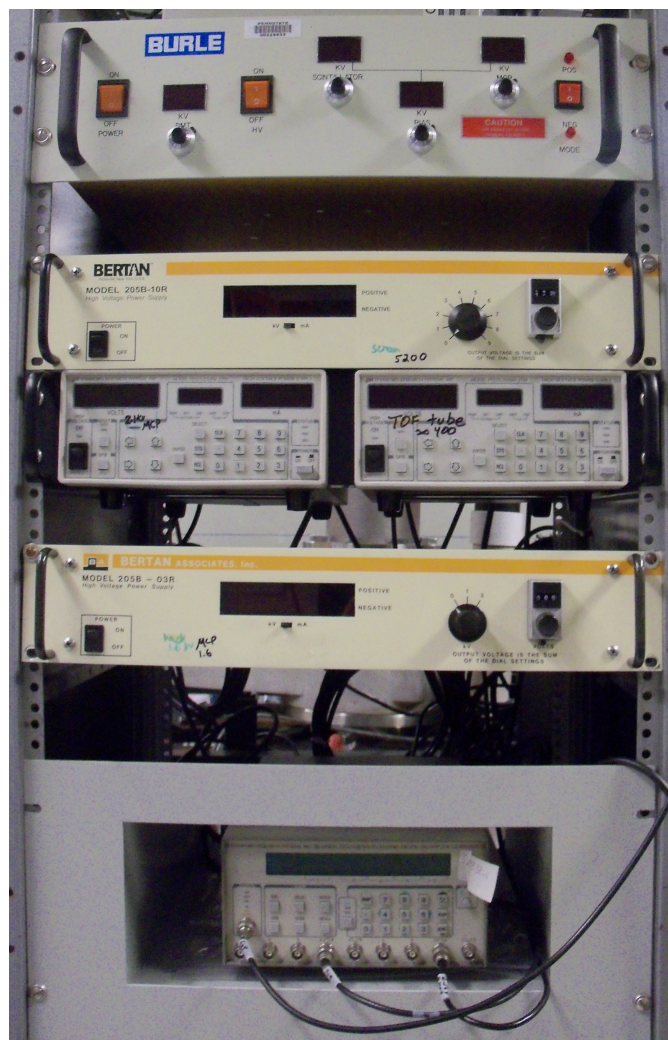
Figure 3.9 The stack of power supplies and timing generators. From bottom to top: the timing generator responsible for gating the repeller and microchannel plates, the power supply for the microchannel plate (+1600 V), the power supply for the pulsed portion of the microchannel plate (left, +2100 V) and the power supply for the flight tube (right, +420 V), the power supply for the phosphor screen (+5200 V), and the power supply for the anion detector.
