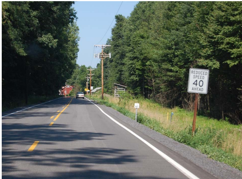
Figure 4 Example of a Transition Zone with a Reduced Speed Ahead Sign
