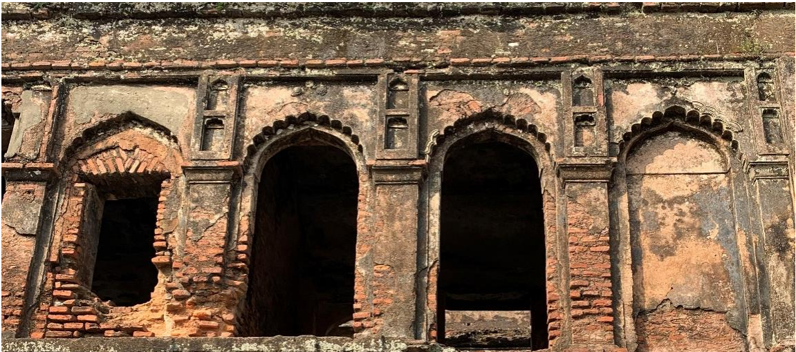
Figure 17: The multiple-cusped arches openings at Panam Nagar, having Mughal influences (Source – Author, 2020)
