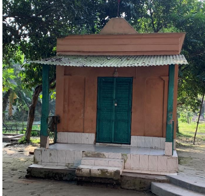
Figure 24: The existing Shiva Temple at Panam Nagar (Source - Author, 2020)
