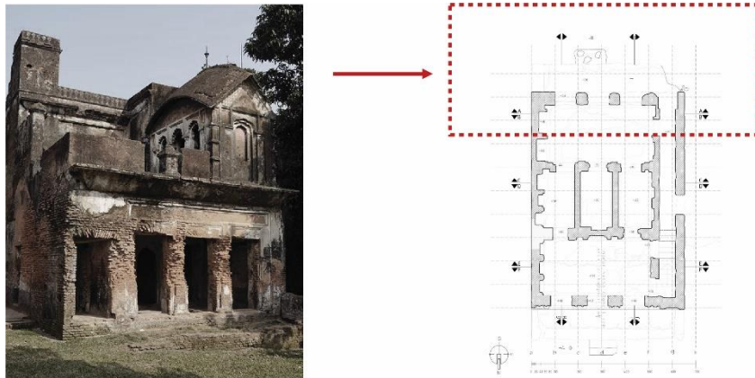
Figure 36: The back facades of the Panam Nagar houses played significant role in the day-to-day life of the inhabitants (Source - Author, 2021)
