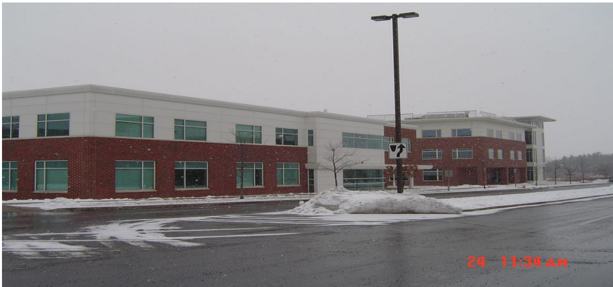
[Figure 4.2, The new Penn State Outreach facility, third home for World Campus]
