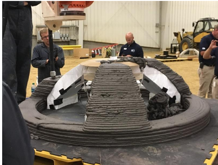
Figure 4-3: Dome printing one arm at a time on the support frame
