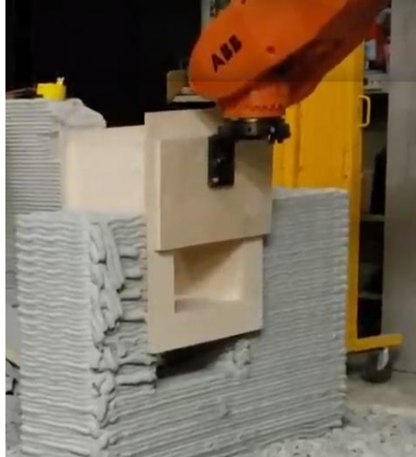
Figure 3-8: Robotically embedding a pre-fabricated structure mid-print
