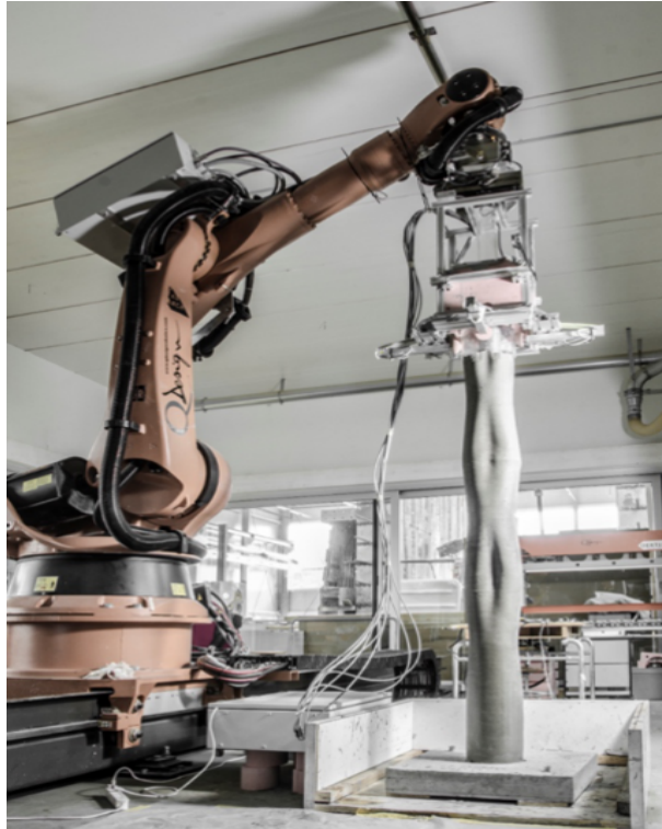
Figure 2.5: Printing a structure by slipforming [5].
