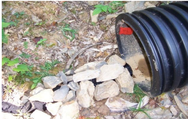
Figure 4.3: Drain pipe (0.5 meter diameter) with a seed trap flush against the lip and disguised with rocks.
