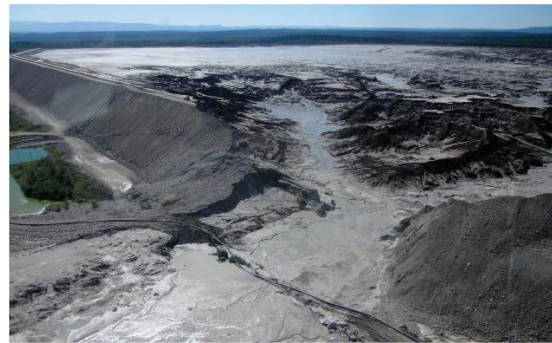
(a) B.C.'s Mount Polley, waste flow into lake (b) B.C.'s Mount Polley, breakage of wall
