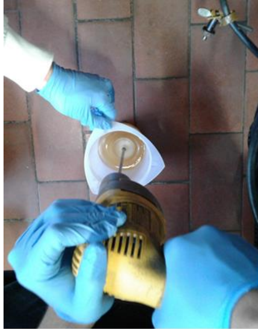
Figure 2-6: Mixing resin with an electric drill.
