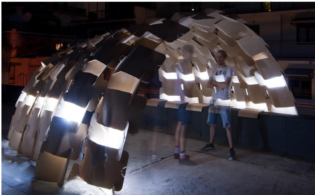
Figure 2-4: Reciprocal frame canopy after construction
