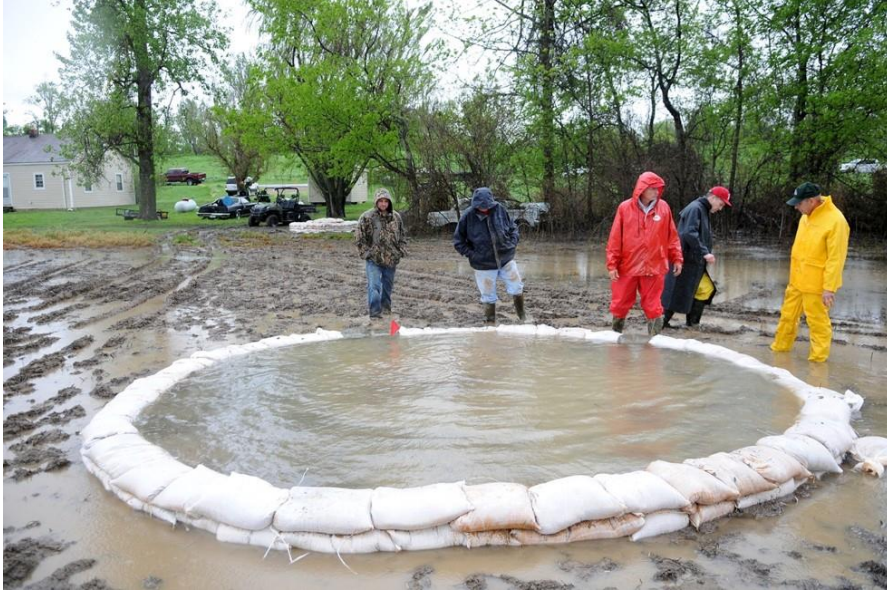
Figure 1-2. Sand bags placed around a sand boil (Hickman, KY, 2011)
