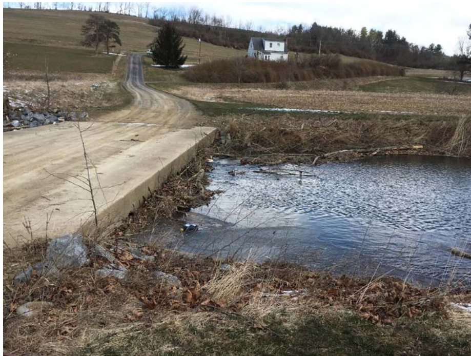
Debris jammed against a farm bridge at a Non-Reference site (Site 234). Residents stated that debris had to be removed frequently to prevent damage.
