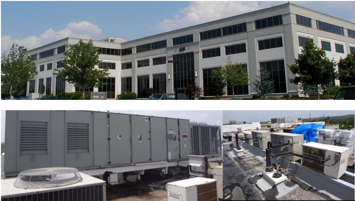
Figure 6-5. Pictures of case study building I.
