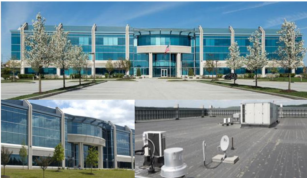
Figure 6-6. Pictures of case study building II.
