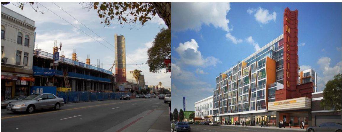
Figure 19: Vida Under Construction (L), Rendering of Completed Project (R) Source: Photograph by Author, Monday afternoon 4:30-5:30 PM; rendering: http://www.vidasf.com
